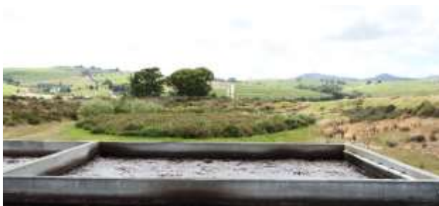
Figure 12. Example of finishing treatment by a bed planted with reeds after a first aerobic floor (Spier Cellar in South Africa)[5].
