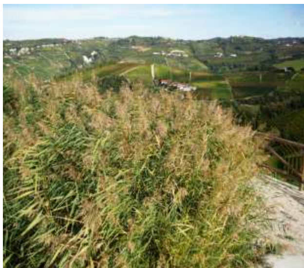
Figure 15. Effluent treatment by a bed planted with reeds on a zeolite support with the Zeofito® device (Baroli cellar in Italian Piedmont)
